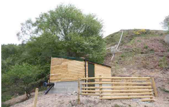
The penstock dropping to the powerhouse.
